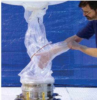
Attach liner then bag out stub
