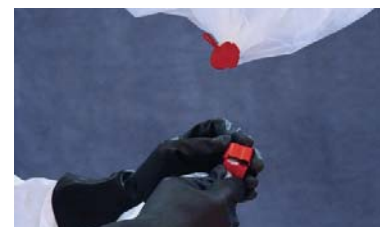
Install crimp cap on crimp body
