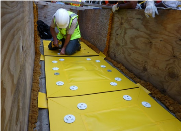
Deploying Flex-Cover™ for water test
